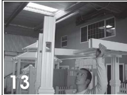
Slide remaining side assembly onto ends of connecting rafters to complete overhead assembly. *for safety and ease assembly we strongly recommend that steps 12 and 13 be done by two people*
