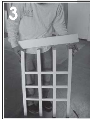
Up-end side grid and cap with top and bottom rails. Repeat steps 1-3 to complete second side grid.
