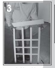
Up-end side grid and cap with top and bottom rails. Repeat steps 1-3 to complete second side grid.
